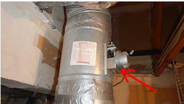
Photo 24-1 Malfunctioning fresh air intake damper.
