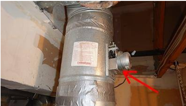
Photo 24-1 Malfunctioning fresh air intake damper.
