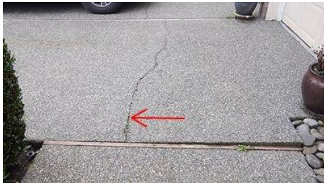
Photo 2-4 Cracked and settled driveway.
