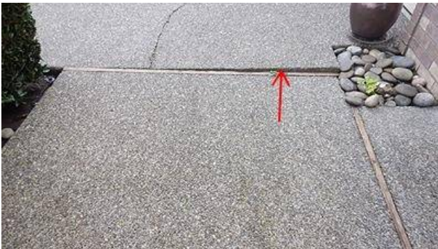
Photo 2-3 Trip hazard at concrete divider.
