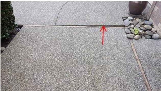
Photo 2-3 Trip hazard at concrete divider.
