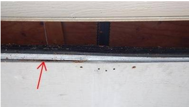
Photo 19-3 Damaged bottom edge of middle garage door.
