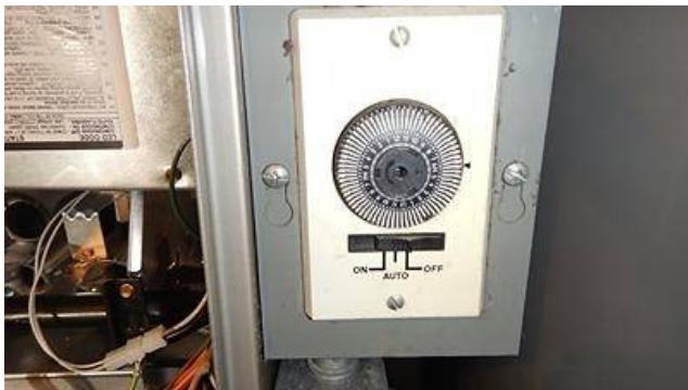
Photo 24-2 Timer control for the fresh air system. The timer is not set for automatic operation.
