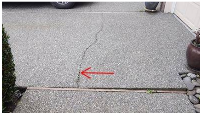
Photo 2-4 Cracked and settled driveway.
