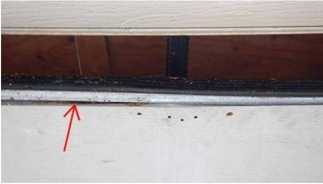
Photo 19-3 Damaged bottom edge of middle garage door.
