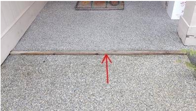
Photo 2-1 Trip hazard at concrete divider.
