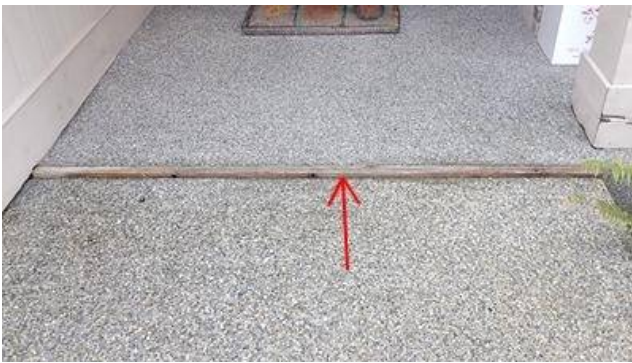
Photo 2-1 Trip hazard at concrete divider.
